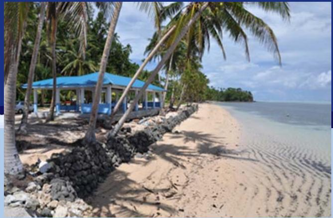
Additionally, the seawall was built out on the beach about 10 feet away from the summer house, and may actually prevent sediment from moving inland close to the building.
